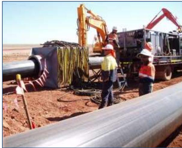
**Figure 6. Reducing the diameter of the PE100-RC liner pipe prior to insertion.**
