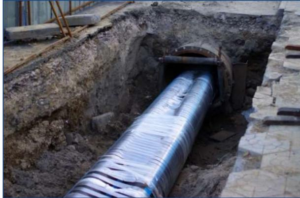
**Figure 7. The pipe folded and strapped being inserted into the old water main**
