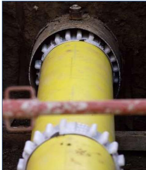
Figure 5. Plastic spacers centralise the PE80 liner in the gas main
